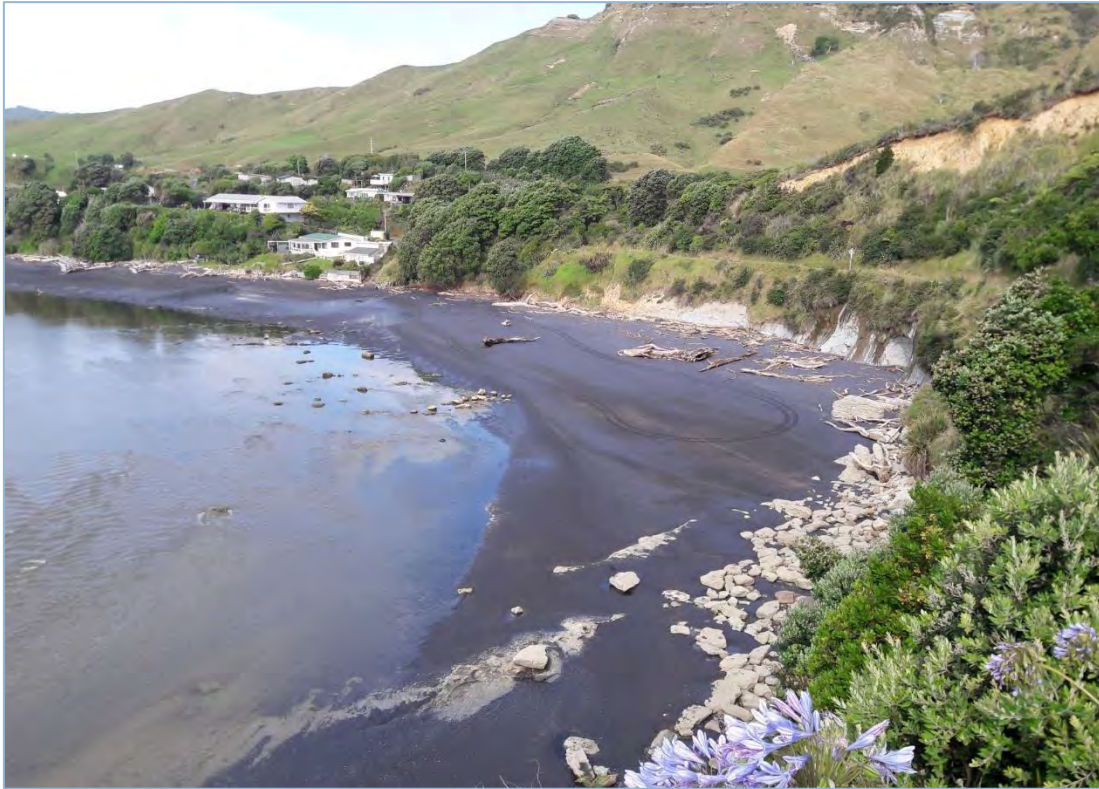
Figure 30: Existing development at Awakino Heads.
