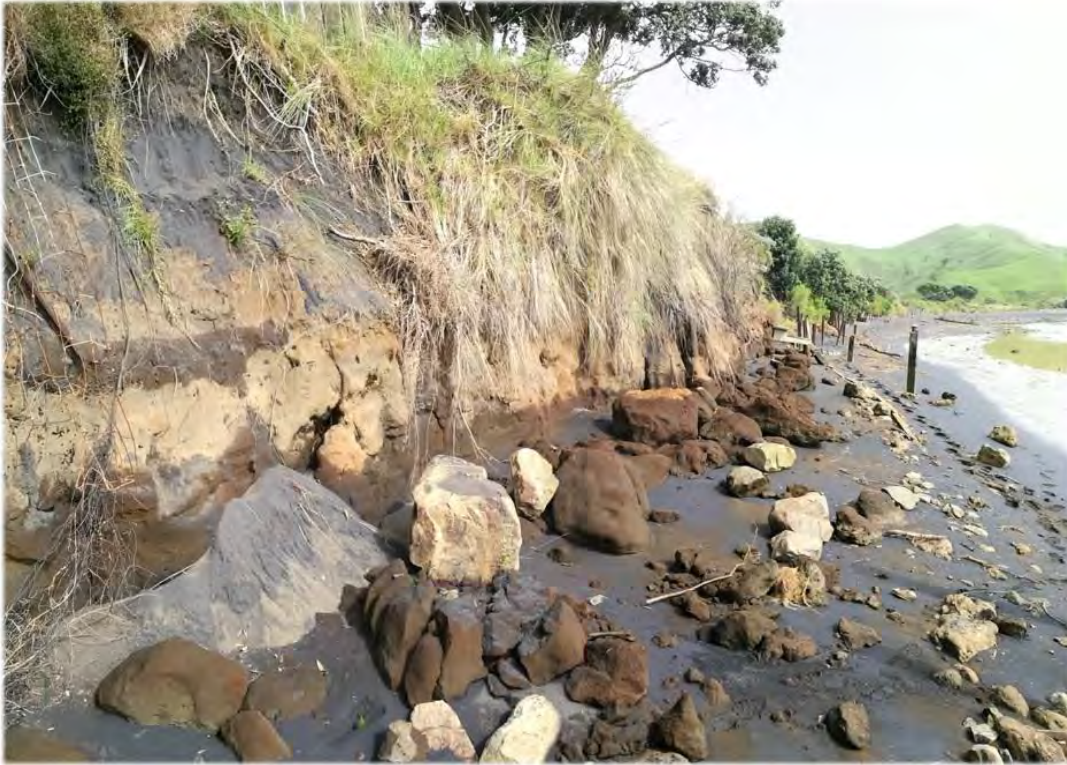
Figure 35: Cemented sands eroding at Marokopa Township.
