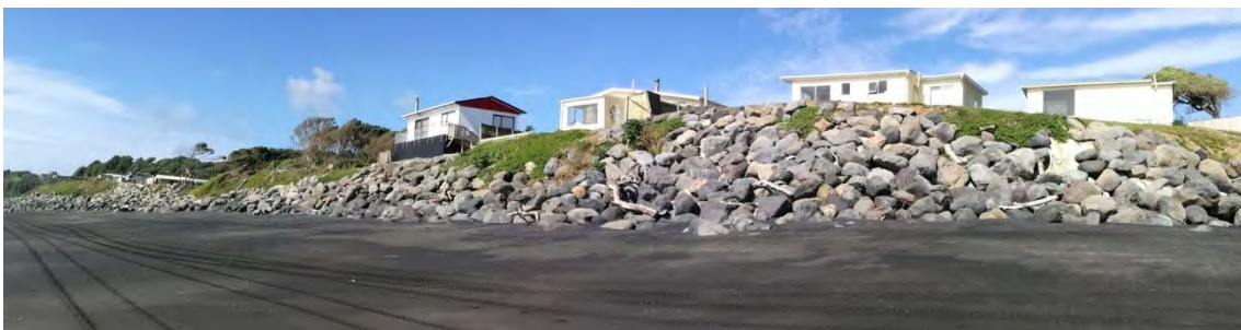
Figure 13: Private seawall fronting Point Road properties, Mokau.
